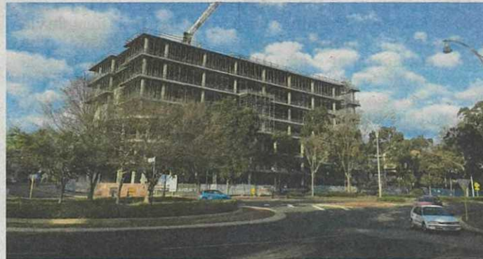
Prime House in Joondalup topped out on August 25.
